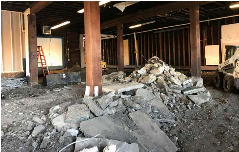
Slab demolition
