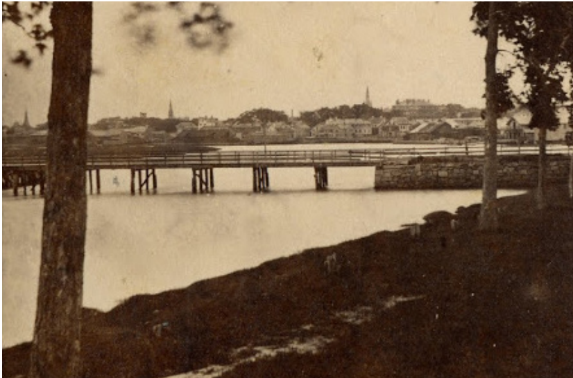
An 1870s view of the Western Avenue Bridge from The Riverside Press
